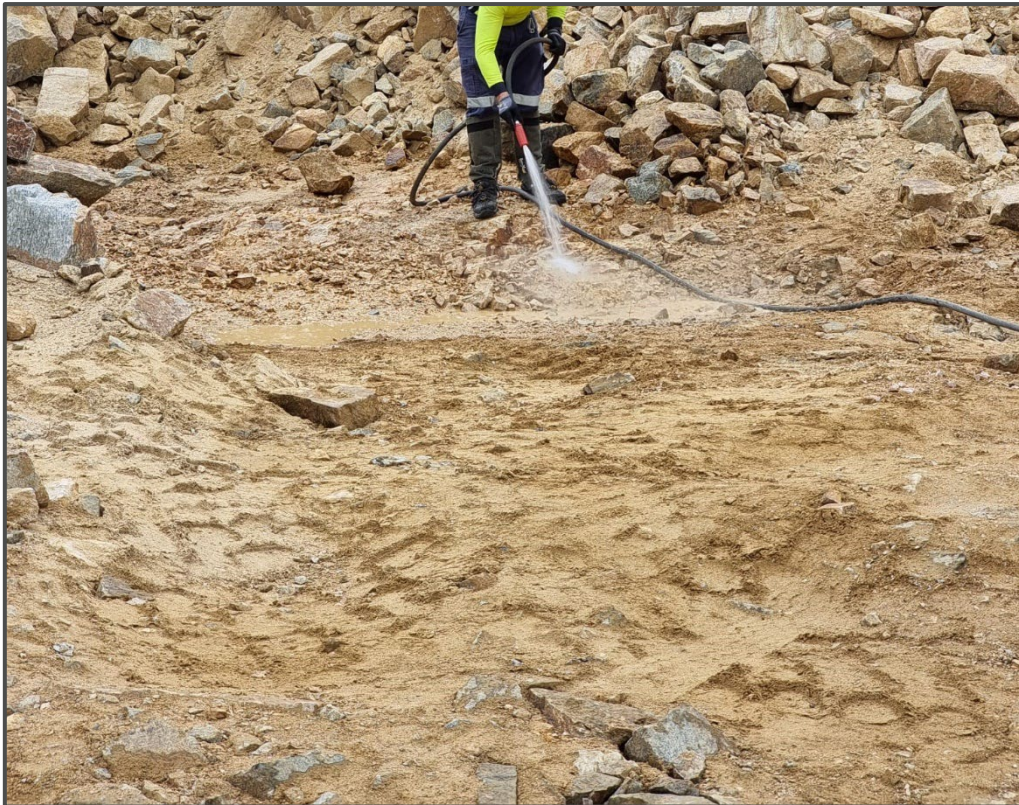
Figure 4: Work underway to expose the natural surface of the Quarry.
