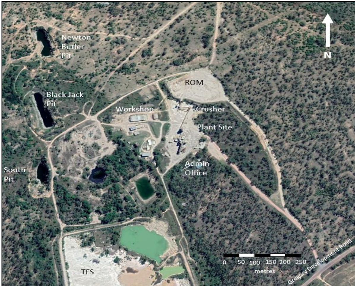
Figure 10: Black Jack site & surface workings
