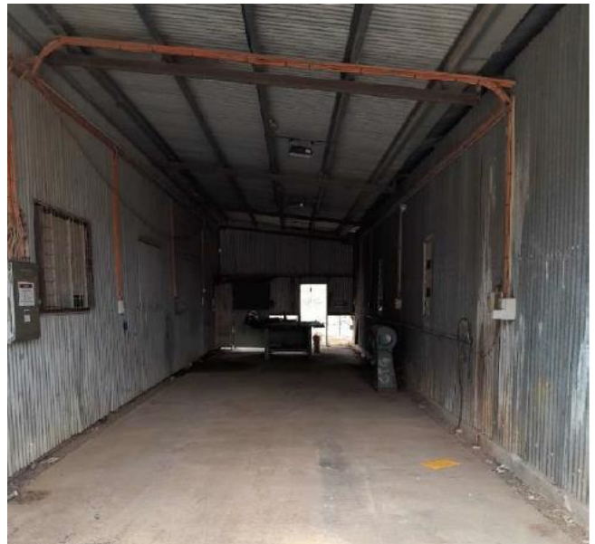
Activated carbon welding bay - after carbon re-bagging
