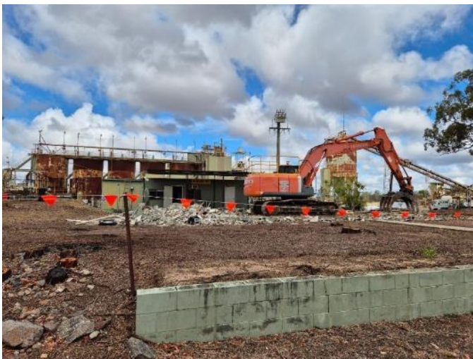
Existing office in poor condition demolished
