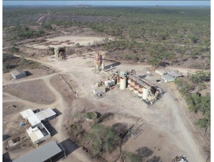
Site after grading and clean-up
