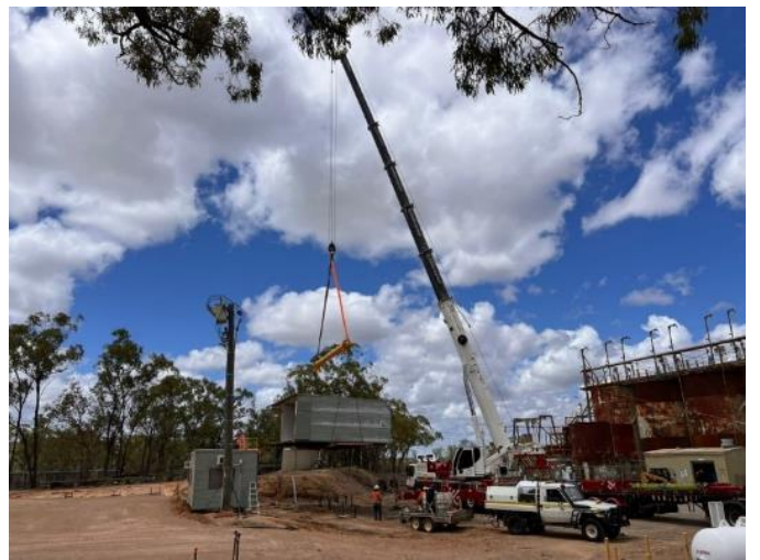
Old buildings in poor condition removed
