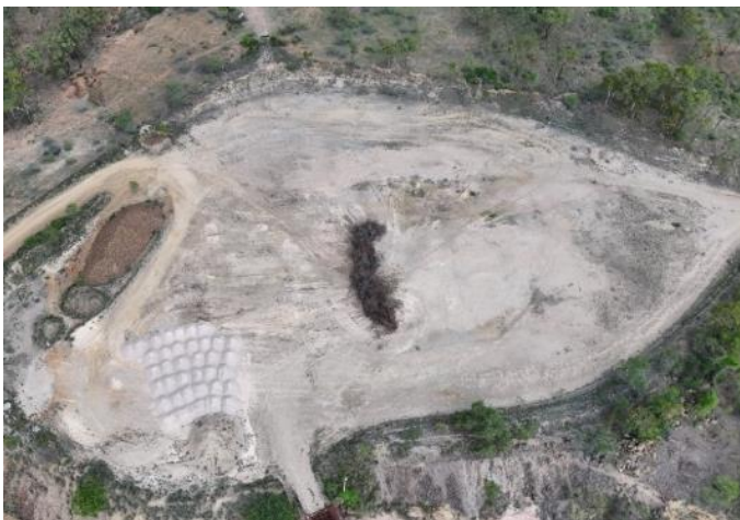
ROM Pad with Discharged Fine Ore
