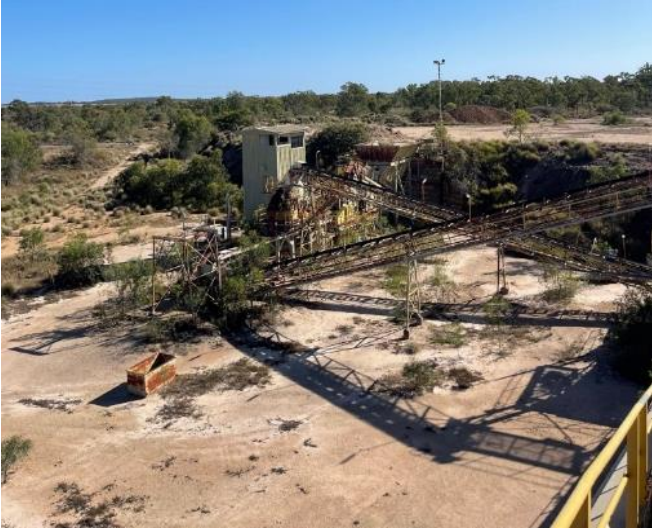
Site before cleanout
