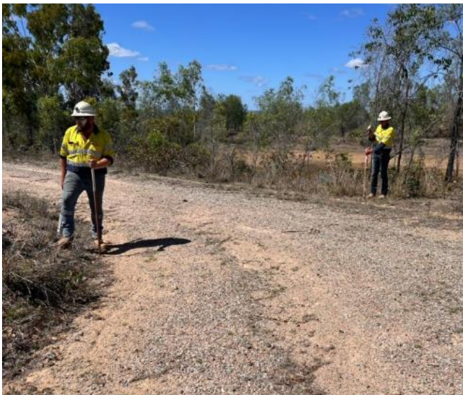
Perimeter fenceline pegging
