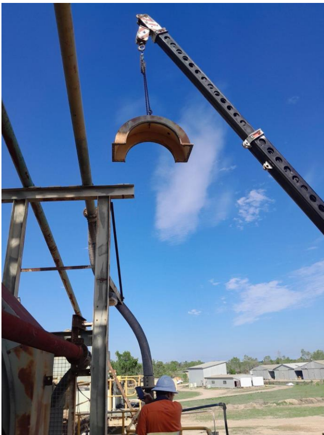
Remove Casing for Ball Mill for Inspection
