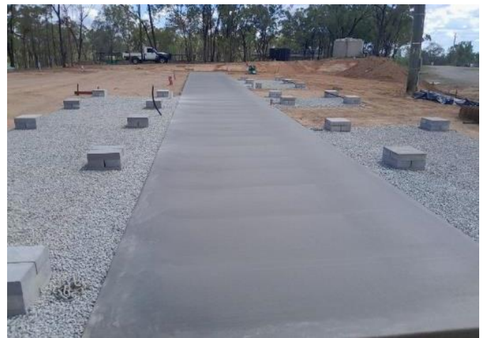
Walkway concreting in progress
