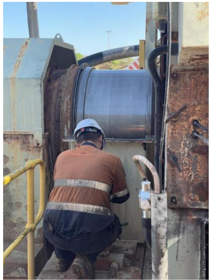
02-BM-01 Ball Mill Bearing Inspection
