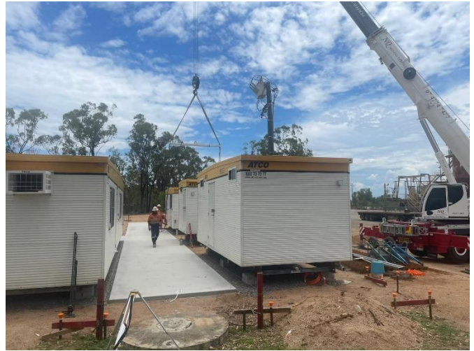
Install and Tie Down NMR ATCO Buildings
