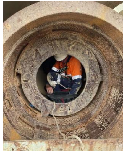
02-BM-01 Ball Mill Liner Profile Inspection and Measurement
