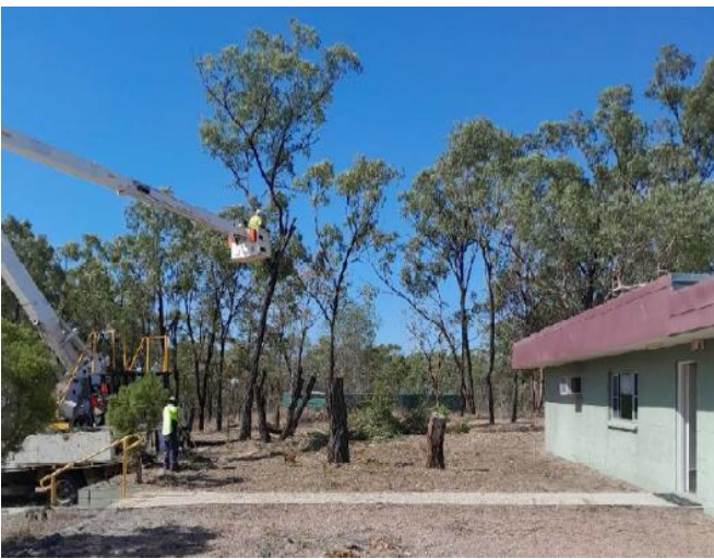
Tree removal at front of administrative area
