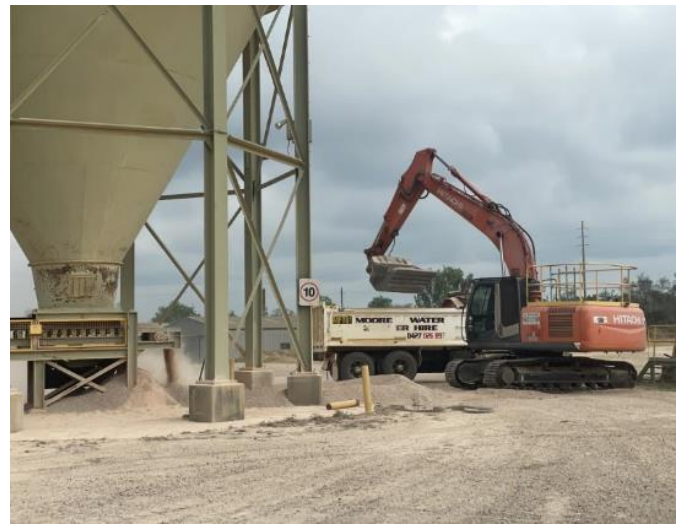
Emptying 900T Fine Ore from 01-BN-02 Fine Ore Bin
