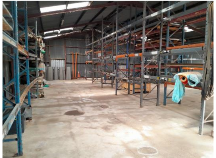
Warehouse after housekeeping and washout
