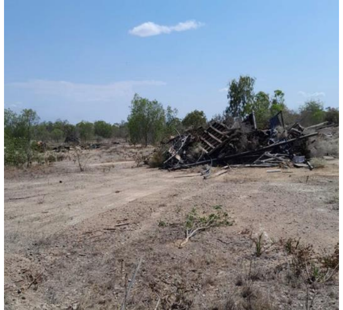
Blackjack Plant workshop area after cleaning
