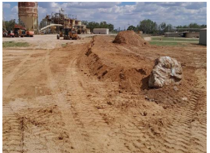
Reinstated bund wall
