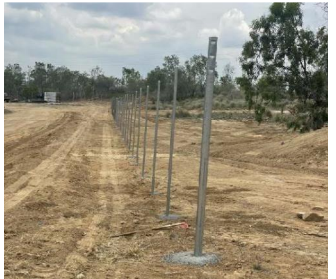
Fence post installation
