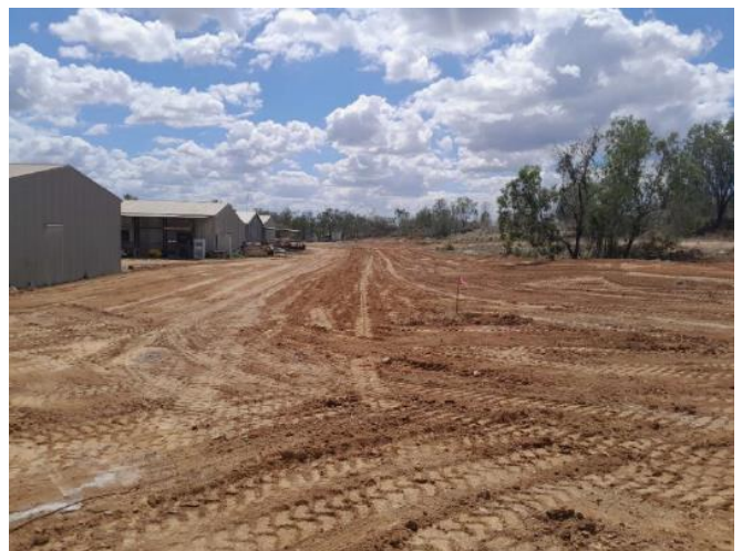
Back of Blackjack Workshop after earthwork
