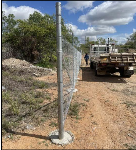
Commence Chain Mesh Install
