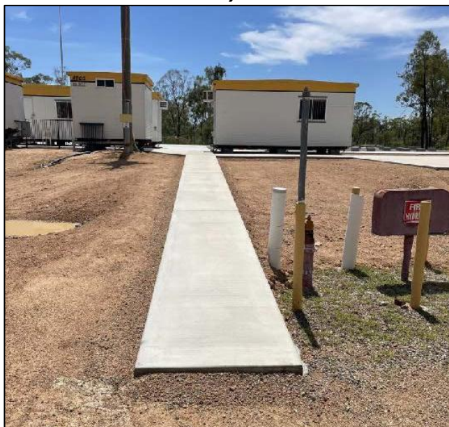
Concrete Pathway to Admin Area
