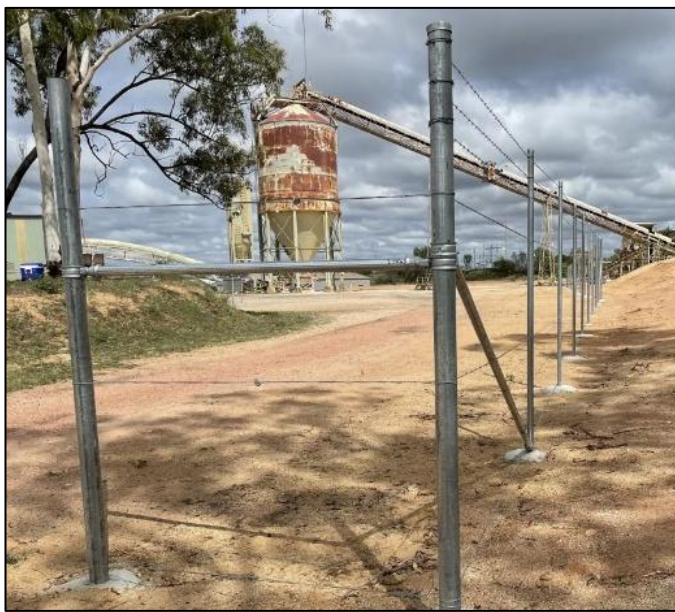
Fencing Wire Installed
