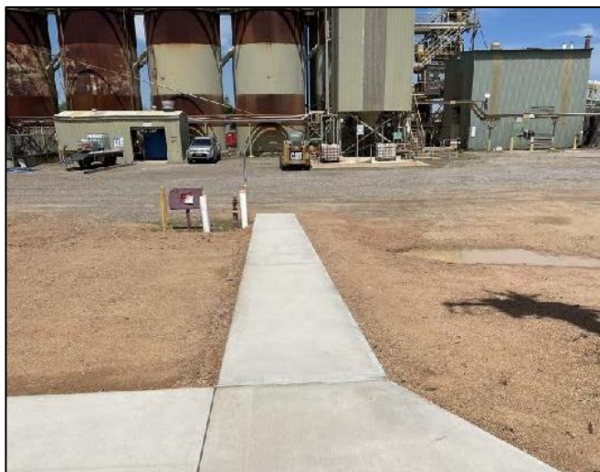
Concrete Pathway to Process Plant
