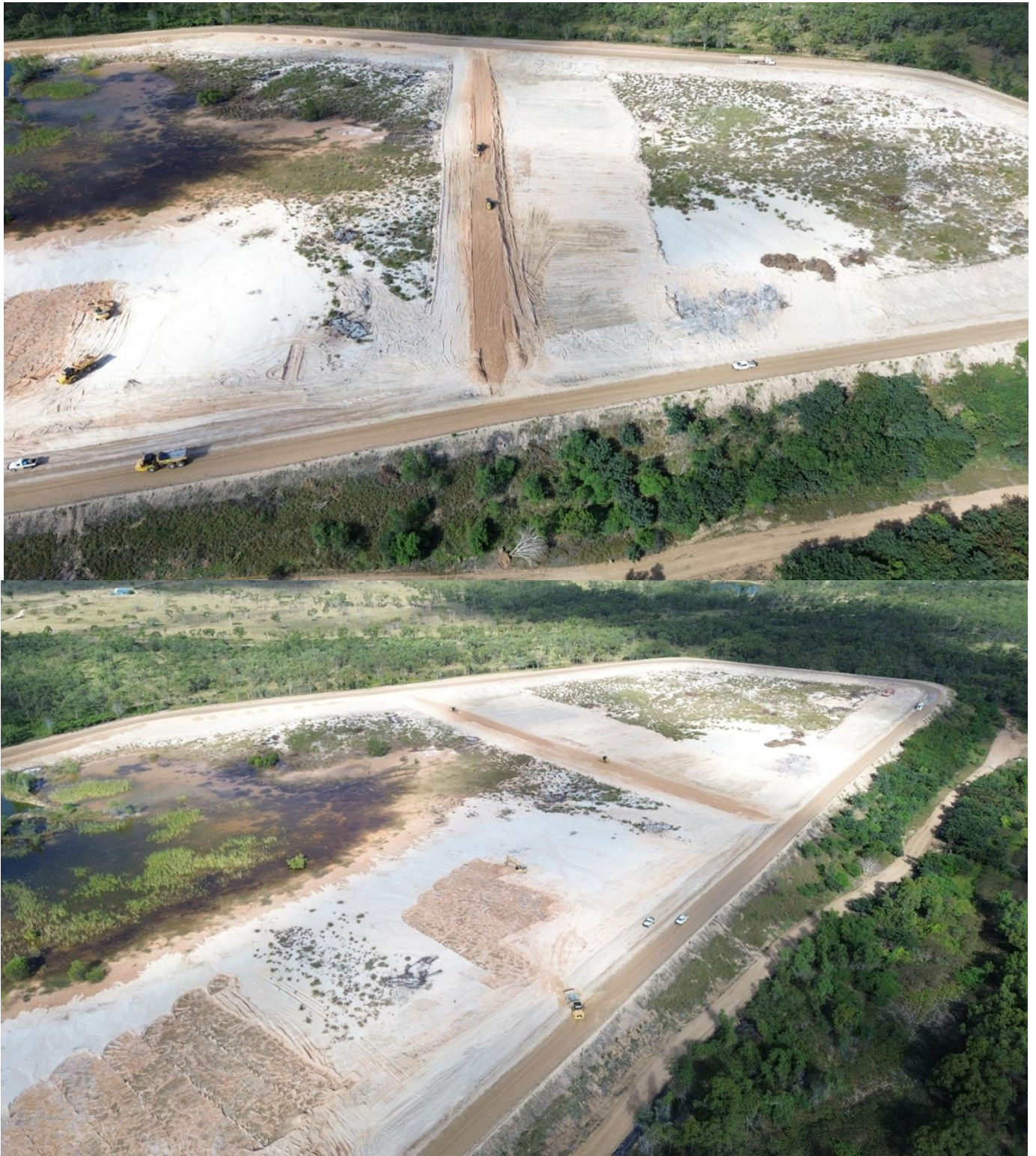
TSF Temporary Bund Wall Separating Northern and Southern Cell
