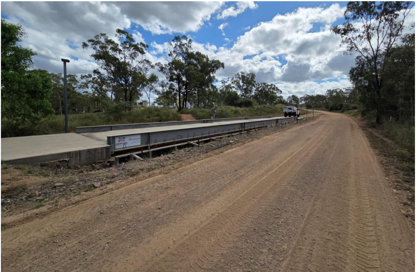
Fully Commissioned and Functioning Weighbridge
