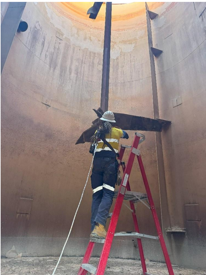
CIL Agitator Blade Replacement
