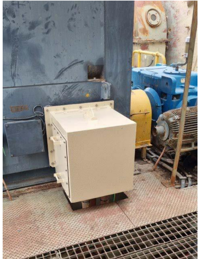
Installation of the Newly Fabricated and Painted Ball Mill Motor Terminal Box
