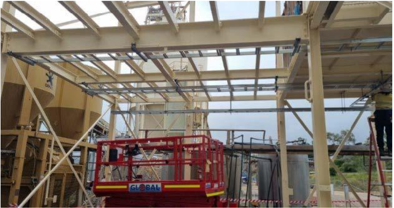
Installation of Cable Tray at Goldroom
