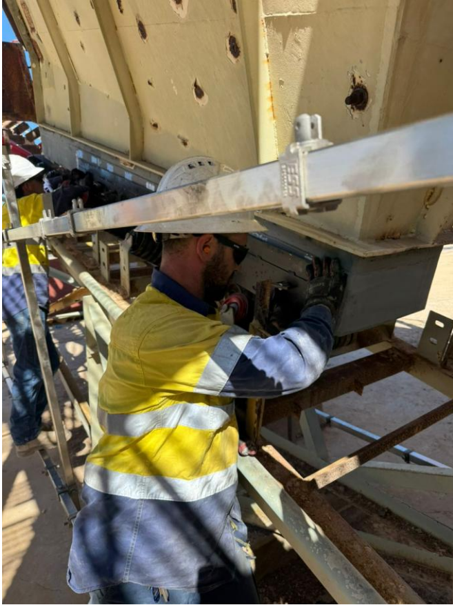
Install New Skirting along CV01
