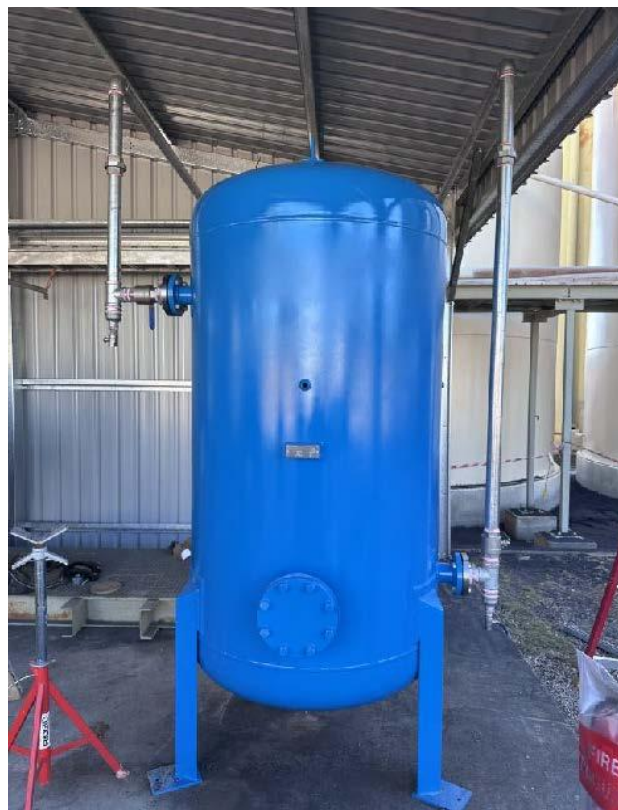
Upgraded and upsized new air receiver
