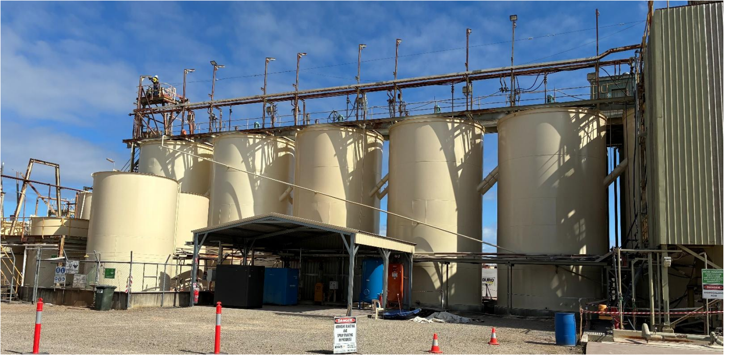
Completed blasting & painting all 6 CIL Tanks
