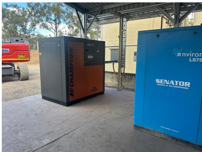
Air compressors installed, ready for Hitachi commissioning
