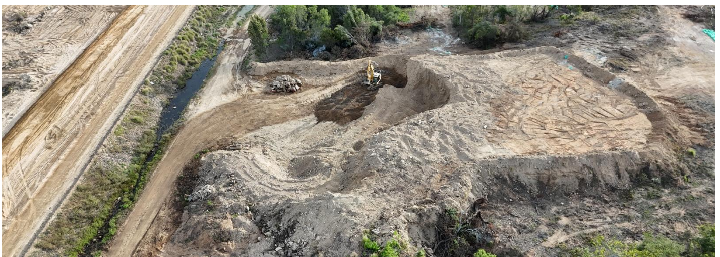
Mixing and blending gravel at Borrowed Area
