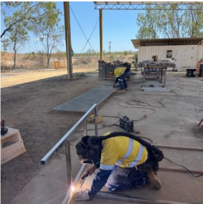
Figure 6c: Ongoing workshop fabrication for overall plant renewal
