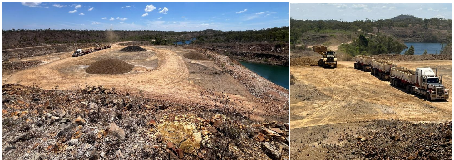
Figure 9c & d: Far Fanning haulage operation
