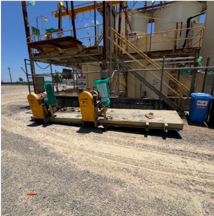
Figure 6e: Removal of previous blower
