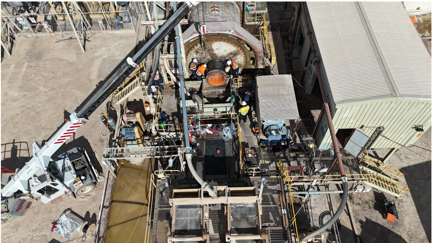
Figure 5c: New white metal lined bearing installation
