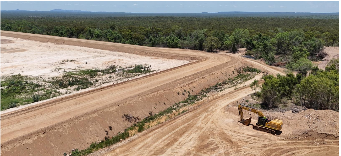
Figure 7c: Blackjack TSF Stage 3 Lift – 7 th layer on Lot 2 & 3
