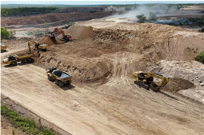
Figure 7a: TSF material stockpile – moisture conditioning
