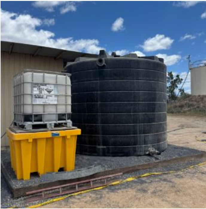
Figure 6a: New cyanide disposal setup at laboratory
