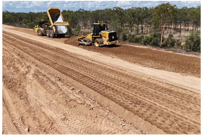
Figure 7b: Earthfill infill placement
