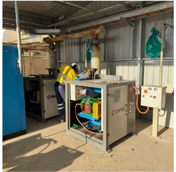
Figure 6f: New blower installation
