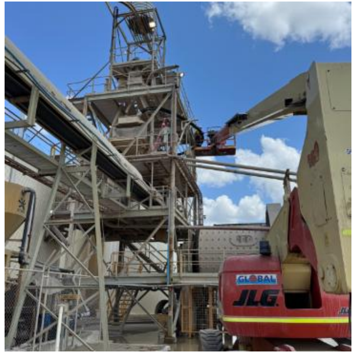
Figure 6b: New mine hose installation
