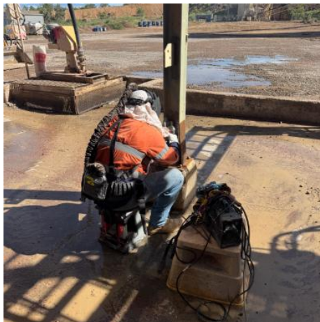
Figure 7: Steelwork repair across site
