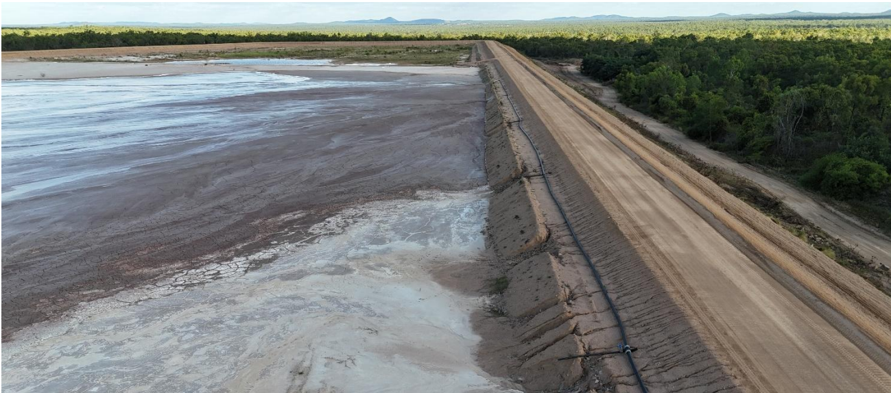
Figure 5: Current TSF with Stage 3 Lift Completed providing tailings capacity till Q3 2027
