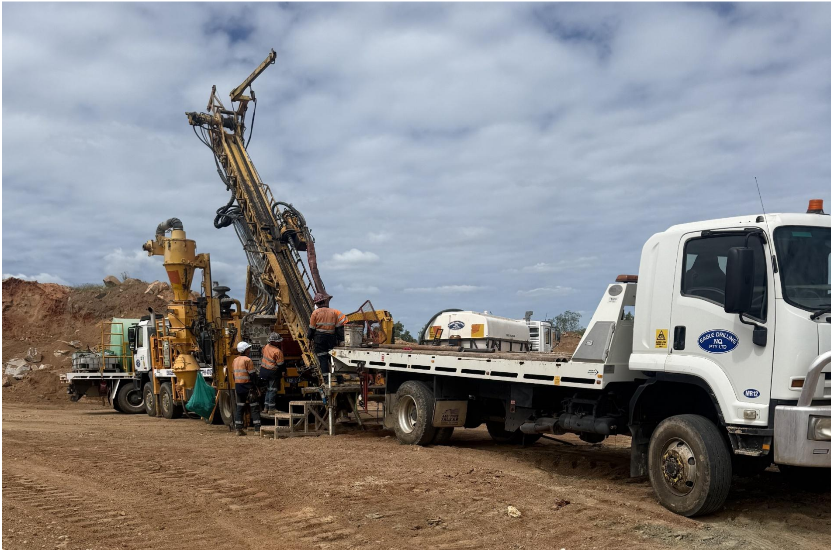
Figure 7: Diamond drilling North Central pit.
