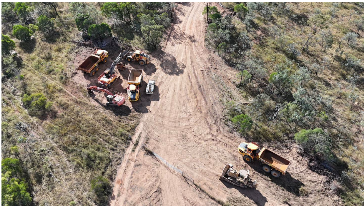
Figure 2: Mining fleet mobilised at Podosky (22 April 2026)
