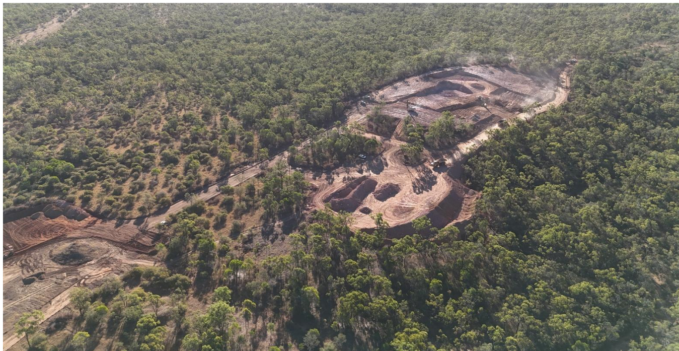
Figure 3: Aerial photograph of the Podosky mining operation highlighting the active pit, ROM pad and Waste Rock Dump area, with mining activities advancing in accordance with the planned development schedule.
