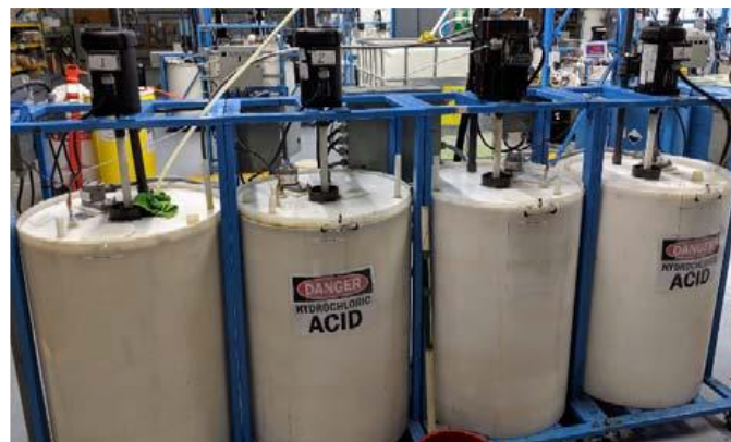
Figure 2 – Batch vanadium reactors in operation at the Company’s Montreal facilities
