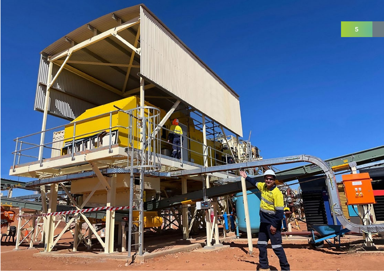
Ore Sorter: The ore sorting system installed at the Pilot Plant.
