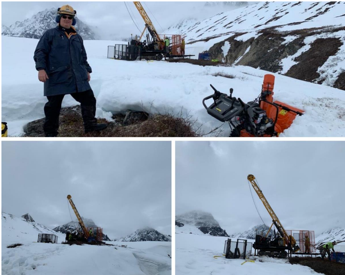
Figure 1. Diamond drill rig set-up at PAD 3 “Starter Pit” Location
