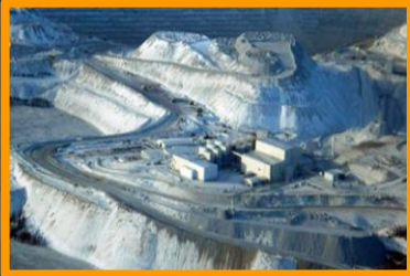
Korbel Central Processing Facility
