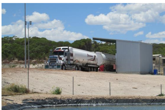
Figure 5 Oil tanker at Jingemia load-out facility
