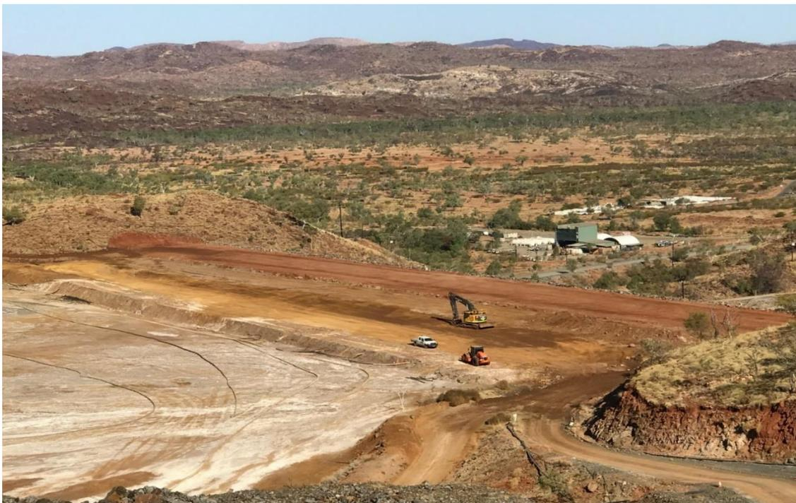
*Earthworks continue on the 3m lift of the tailings storage facility*
