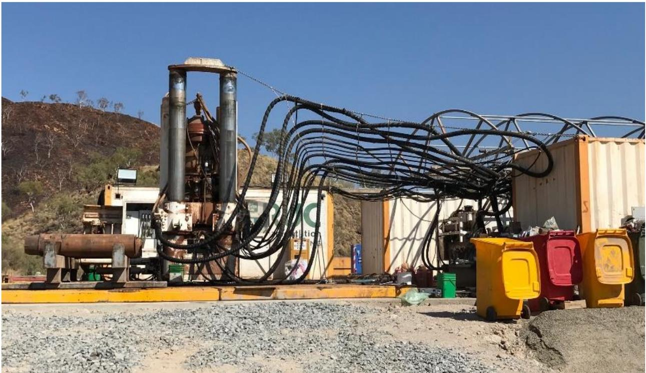
*Raisebore drilling the pilot hole for the ventilation intake rise*
