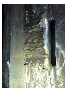
Figure 5. New crack after repair just below the repair job
