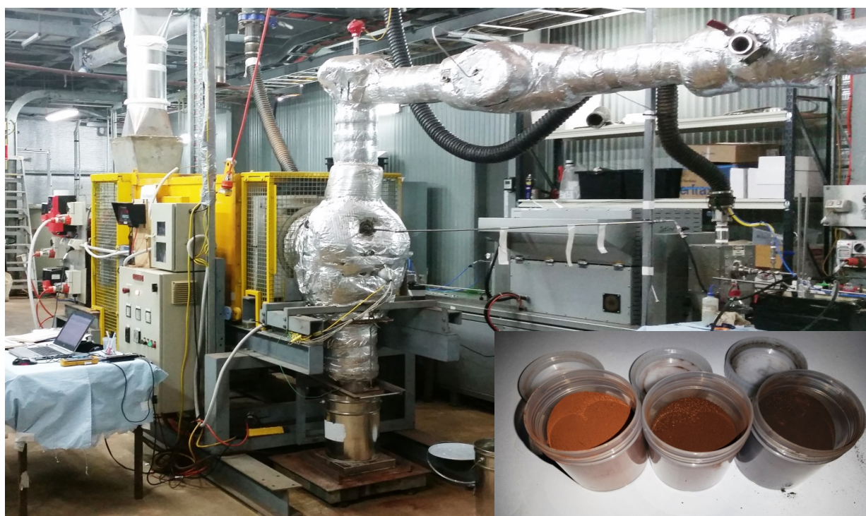
Figure 3: ANSTO Pilot Plant roaster and products at varying temperatures (inset)
