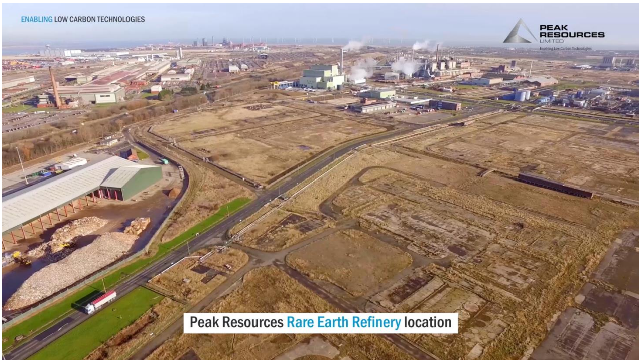
Figure 3 - The Refinery plot in the Wilton International Site
