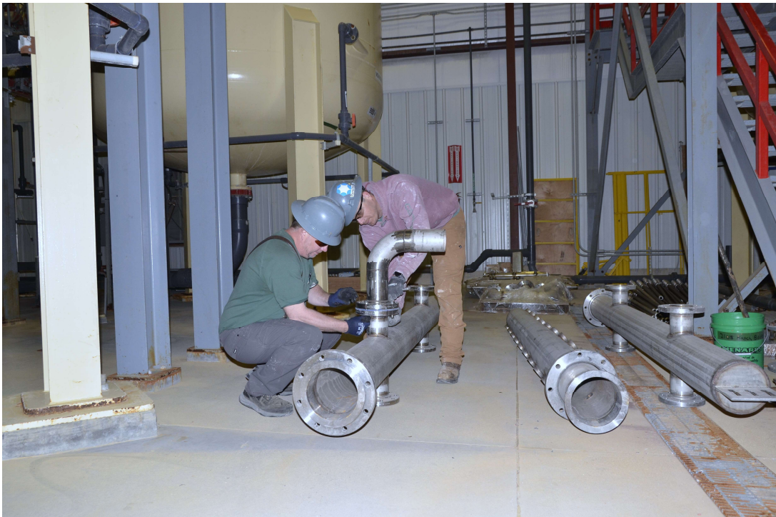
IMAGE 2: Plant transformation construction efforts in-progress
