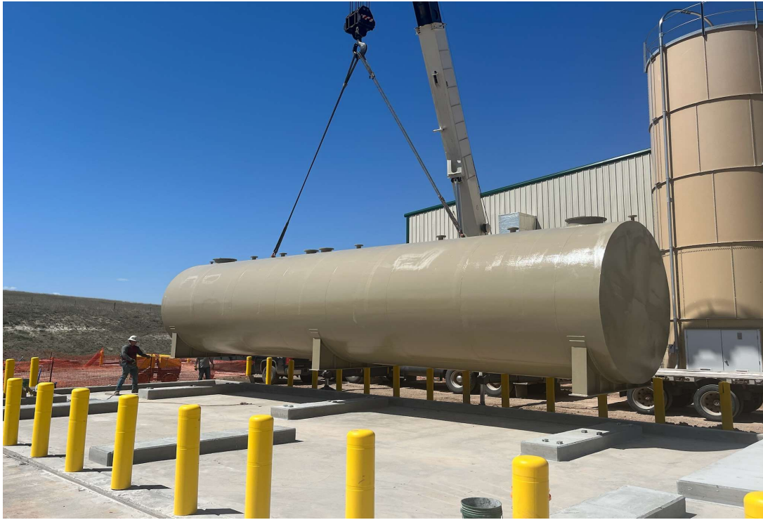
IMAGE 1: Placement of the high-volume sulfuric acid storage tank at Lance
