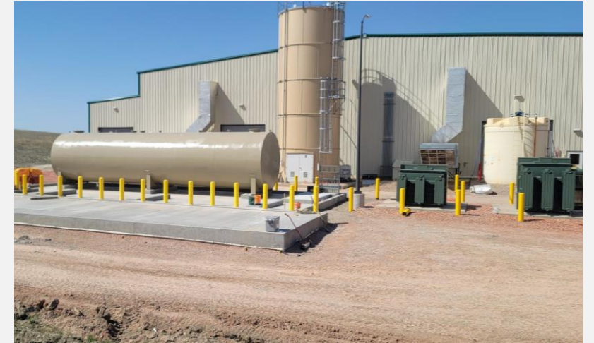
New installation of a high-volume acid storage tank
