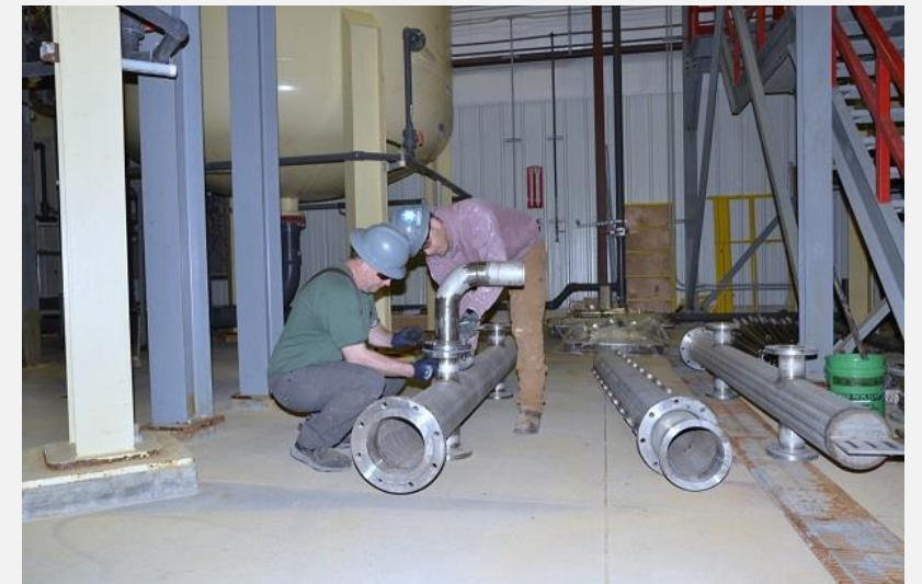
Re-piping of the Process Plant
