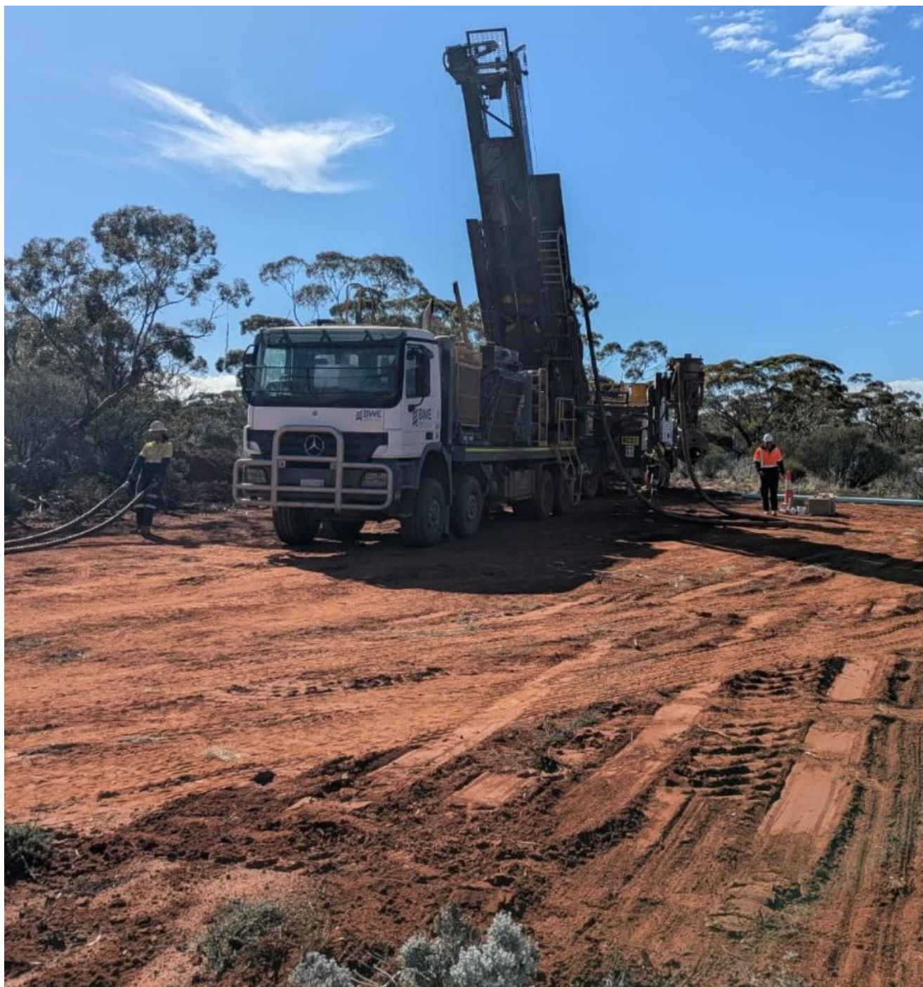
Figure 3. BWE drill rig setting up on hole (26RHRC001).
