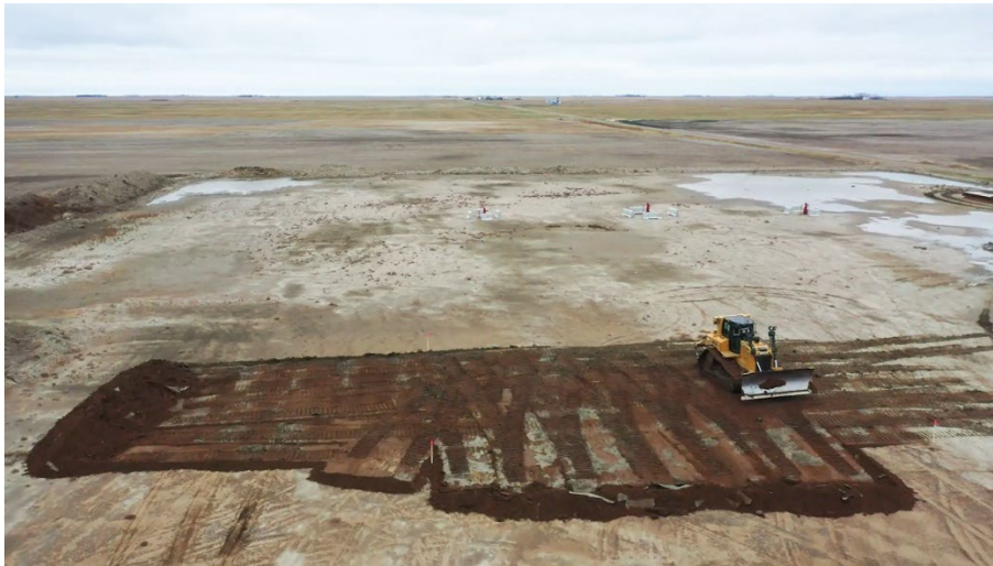
Figure 1: Foundation works on Pad #1
