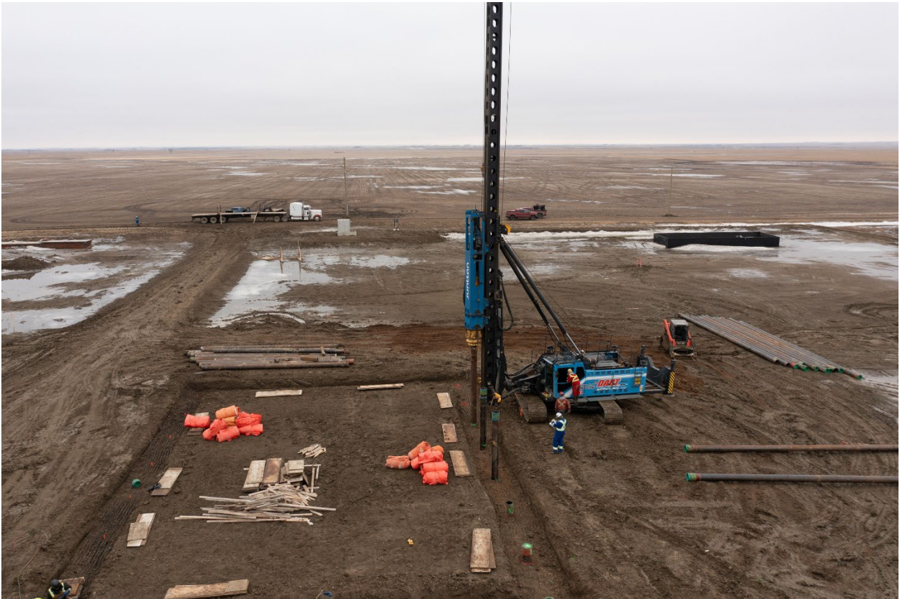
Figure 1: Installing piles for facility foundation at Pad #1
