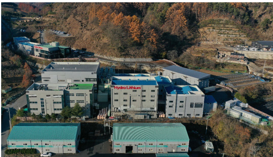
Figure 2: Hydro Lithium Refinery in Korea
