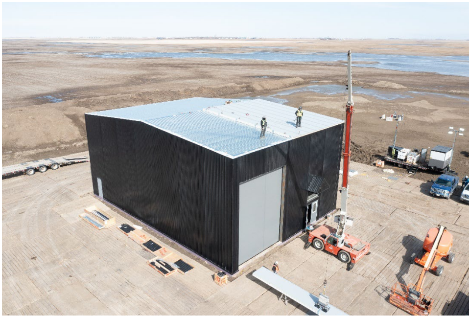
Figure 3: Construction of Prairie Lithium production facility in Saskatchewan, Canada
