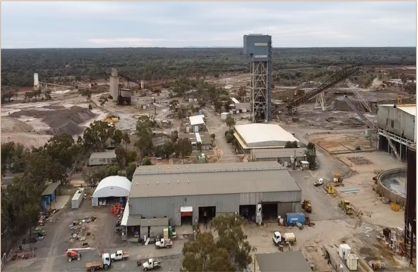
Figure 6: Endeavor surface workshop and headframe – November 2022
