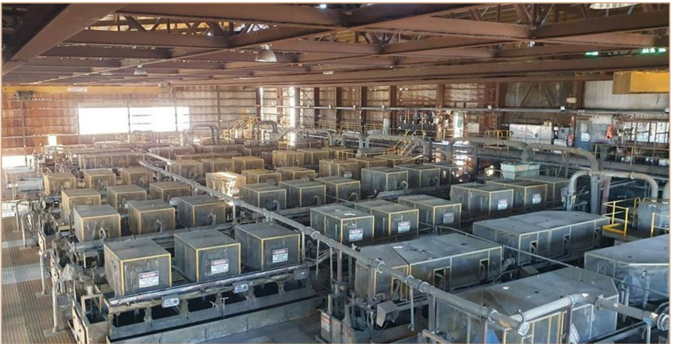
Figure 4: Endeavor – Lead / Zinc Flotation floor (February 2023)
