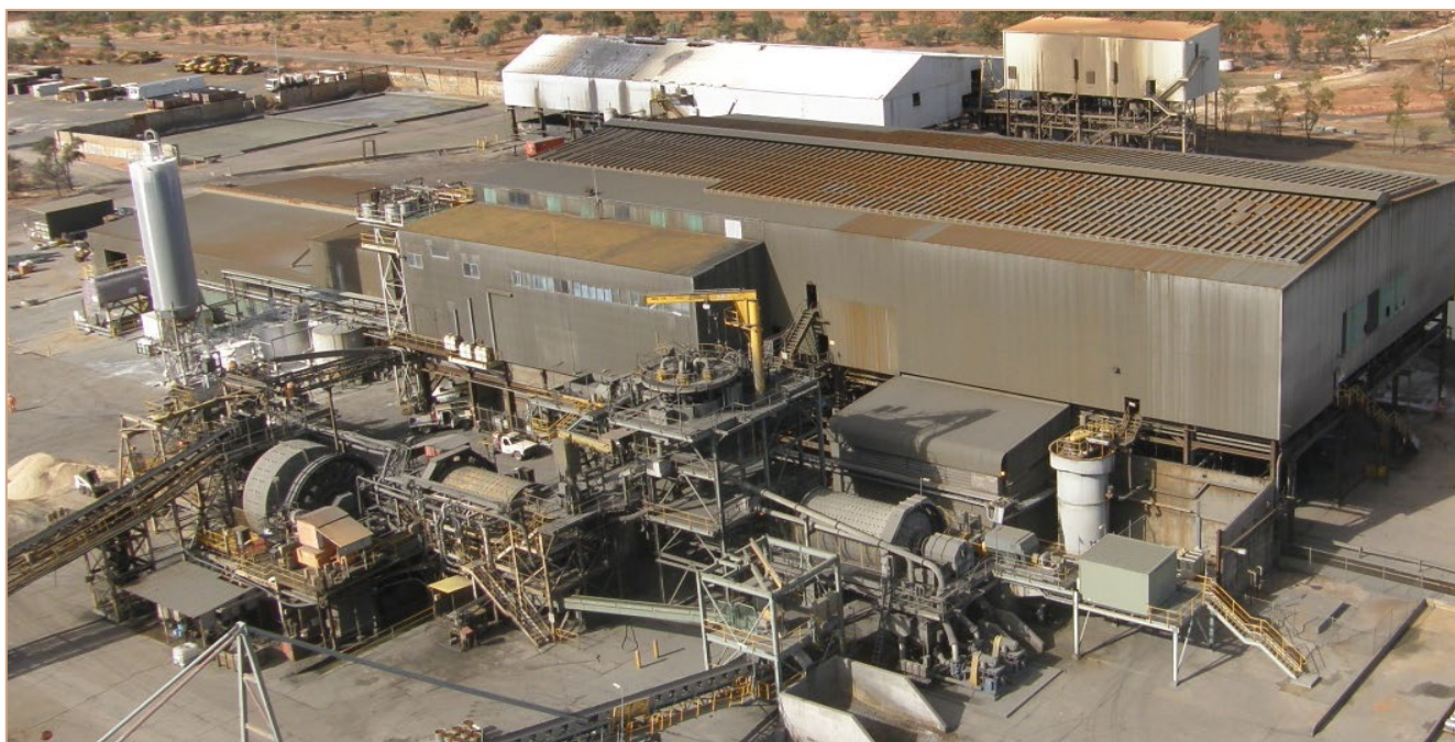
Figure 3: Endeavor Project: 1.2 MTPA Processing Plant (2019)
