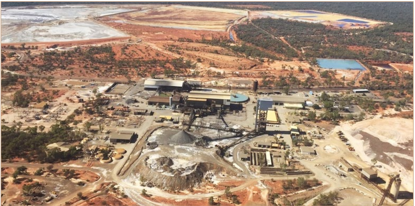
Figure 2: The Endeavor Mine – Surface Infrastructure (2019)
