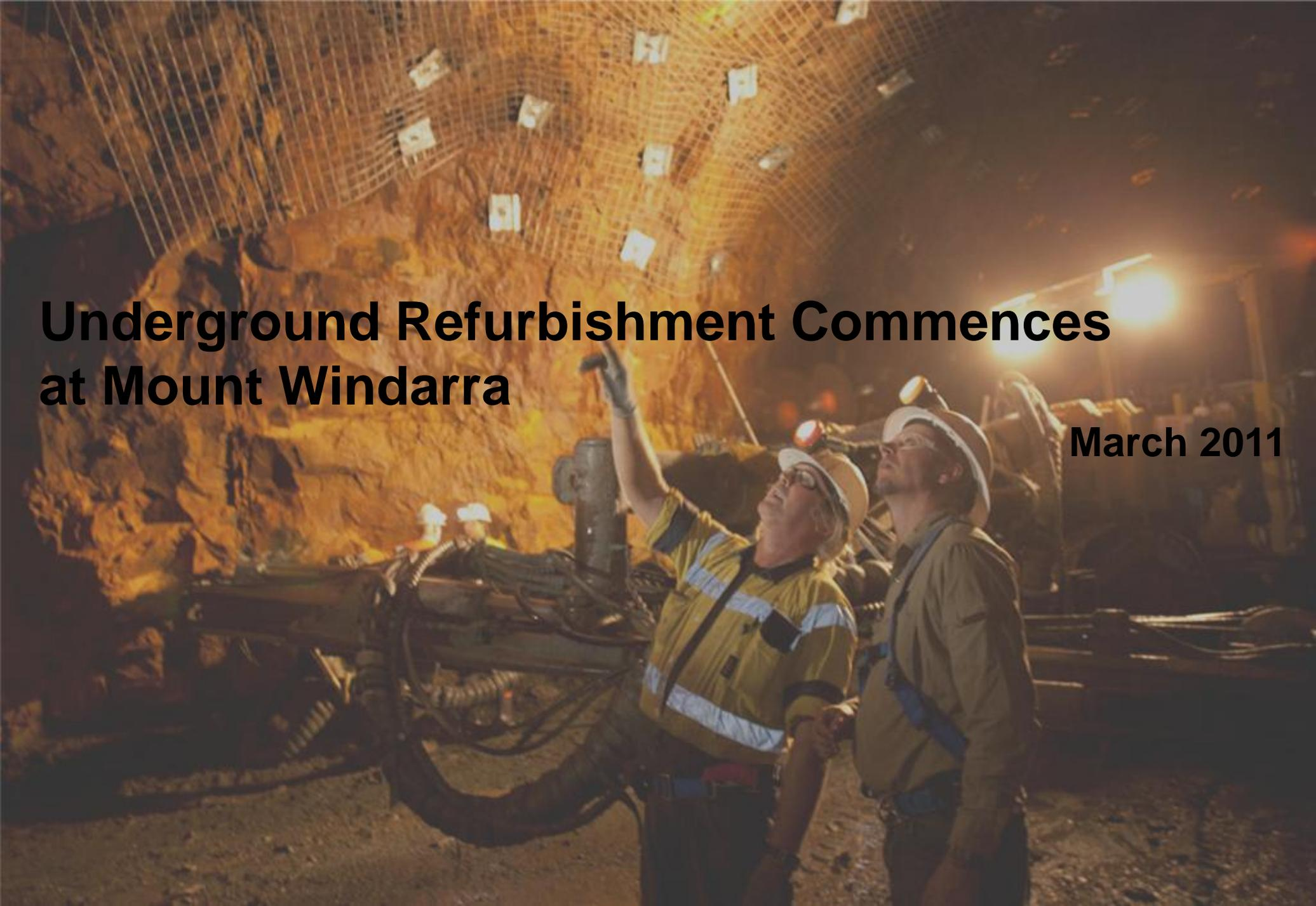
A photograph of an underground mine tunnel under refurbishment. The ceiling is covered in a dense grid of steel reinforcement mesh. Two workers in safety gear are in the foreground, looking up at the ceiling. One worker is pointing upwards. The scene is dimly lit with warm, yellowish light from overhead fixtures. Various cables and equipment are visible in the background.
