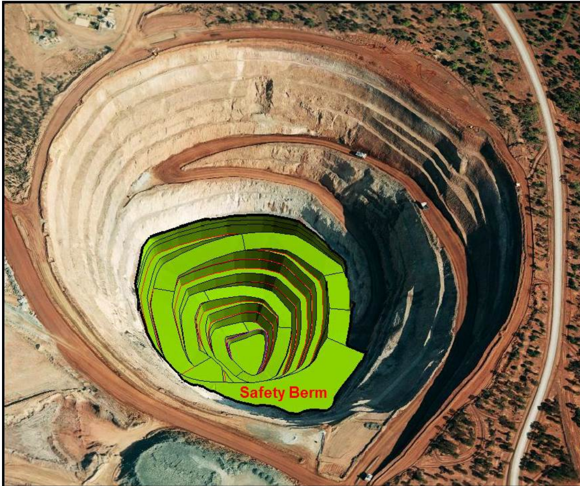
Figure 2: Revised Black Swan Pit Design (oblique view) to Account for Slip on the South Wall
