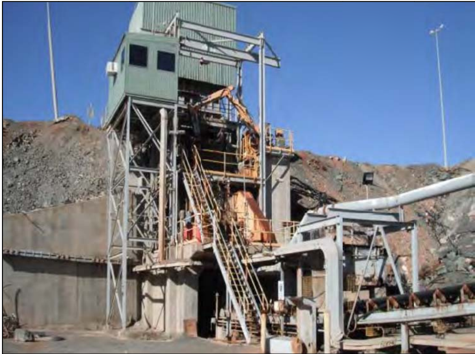
Figure 3: Black Swan primary crushing circuit
