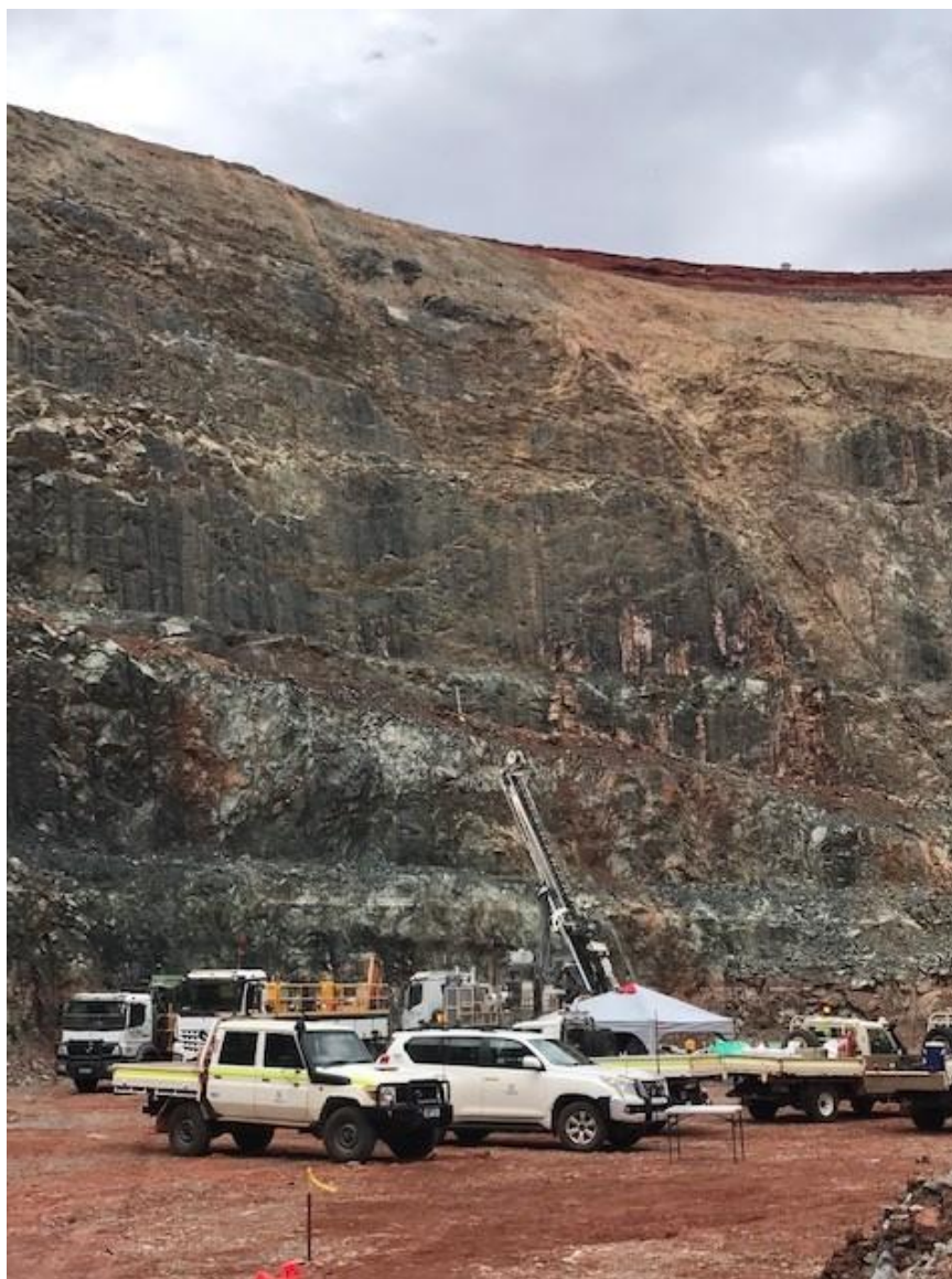
FIGURE 1 – DRILL RIG OPERATING IN THE BLACK SWAN OPEN PIT
