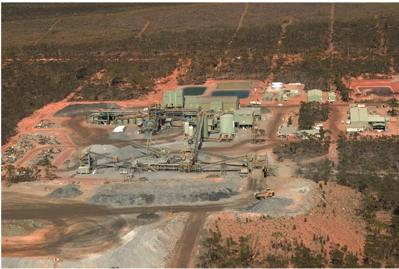
Figure 15: Lake Johnston Process Plant
