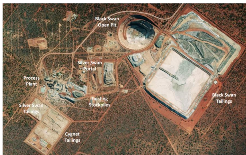
Figure 1: Black Swan Site Map Noting Significant Infrastructure
