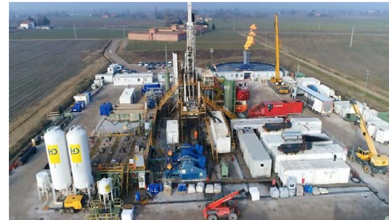
Podere Maiar – 1 well (drilled in Dec 2017)
