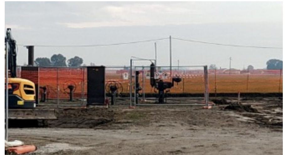
Picture: Podere Maiar – 1 well site in development
