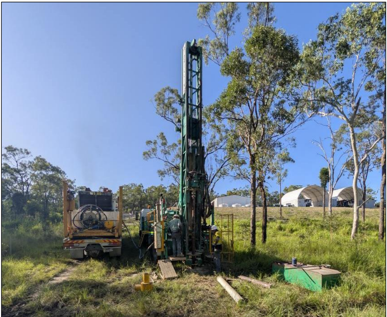
Figure 2: Groundwater monitoring bore being drilled at Mt Chalmers.
