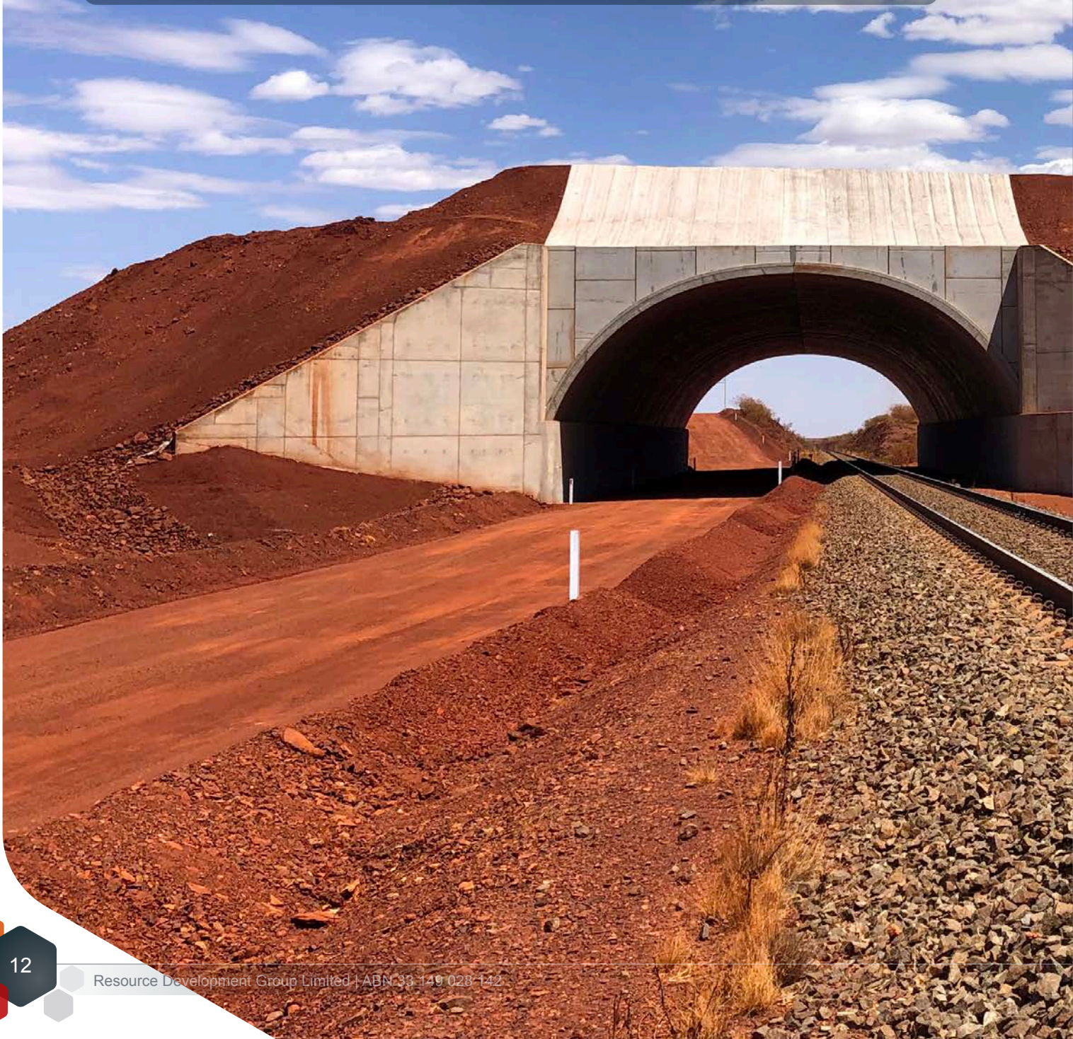
Below: Abrolhos Overpass constructed at Cloudbreak Mine Site, Pilbara region of WA, for Fortescue Metals Group (FMG).
