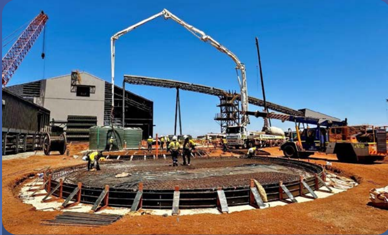
Above: Construction of tank foundations at Onslow Port
