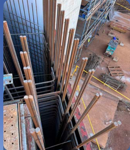
Formwork set up at Ken's Bore project
