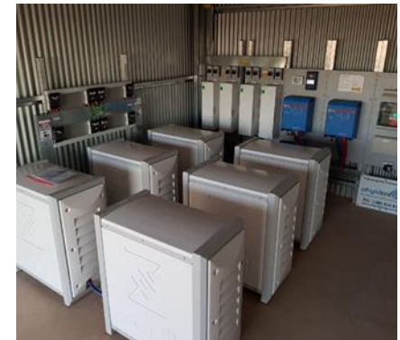
6 x Zcell off-grid installation in SW Queensland
