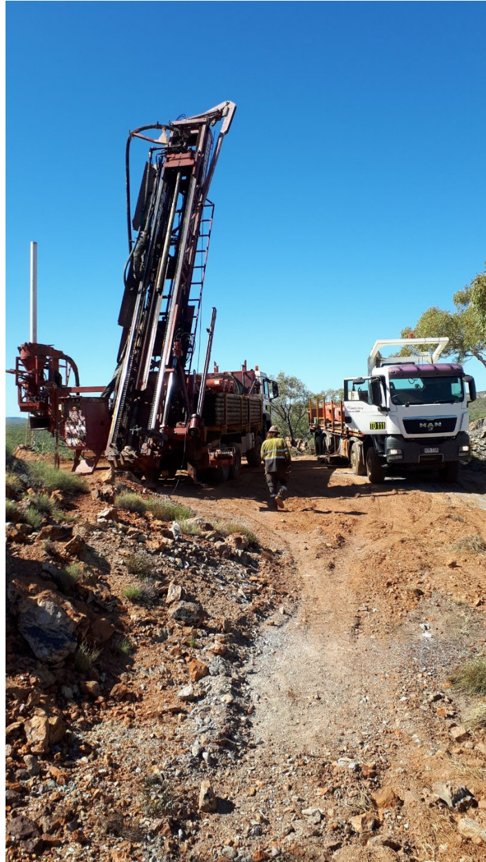
Figure 2: Drilling rig about to commence work
