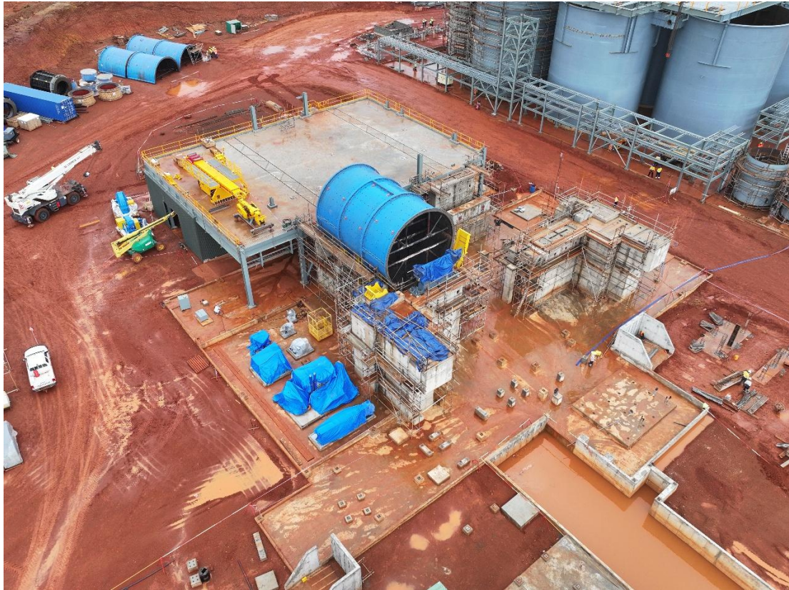
Figure 2: View of Milling building showing mill suspended slab completed and SAG Mill Installation (13 August 2025)
