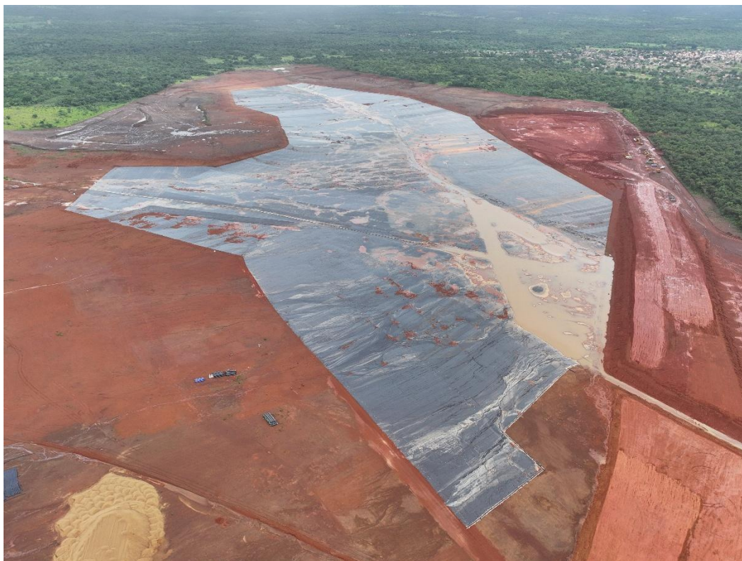
Figure 4: Tailings storage facility showing the extent of lining and main embankment construction (13 August 2025).
