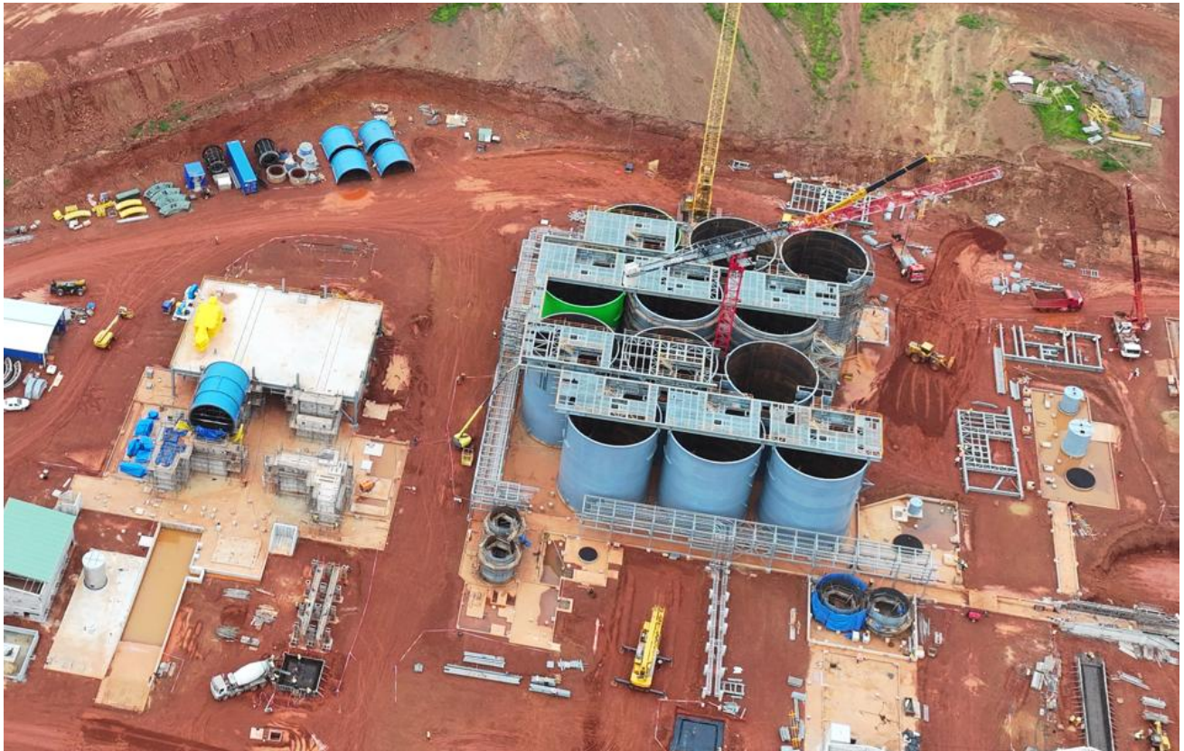
Figure 3: View of CIL with pipe rack and top of CIL tank steel erection (19 August 2025)
