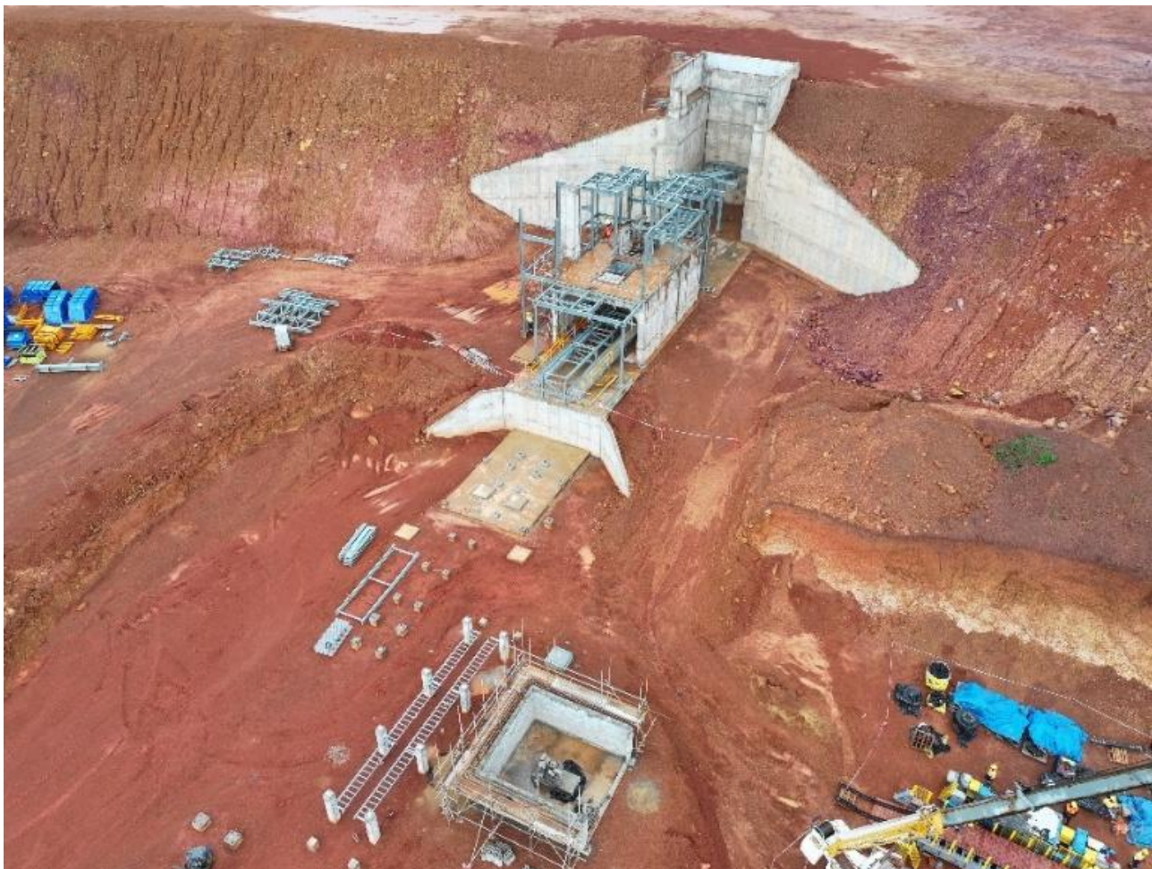
Figure 6: Primary crusher steel erection progress (13 August 2025)
