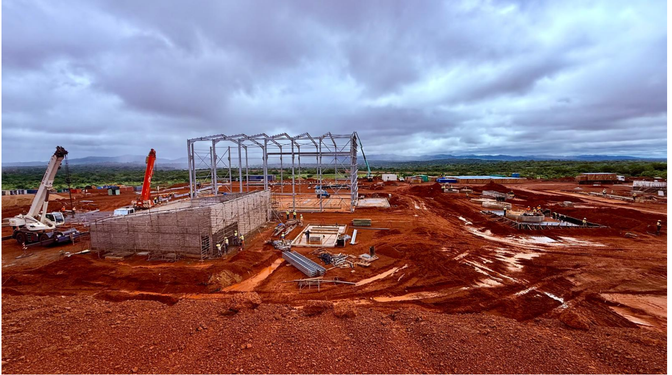
Figure 8: Power Station with steel erection commencing and switch room nearing completion (13 August 2025)
