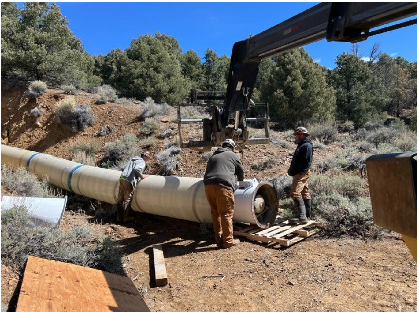
Photo 1 – Vent assembly and installation - Superior Level 4 Adit
