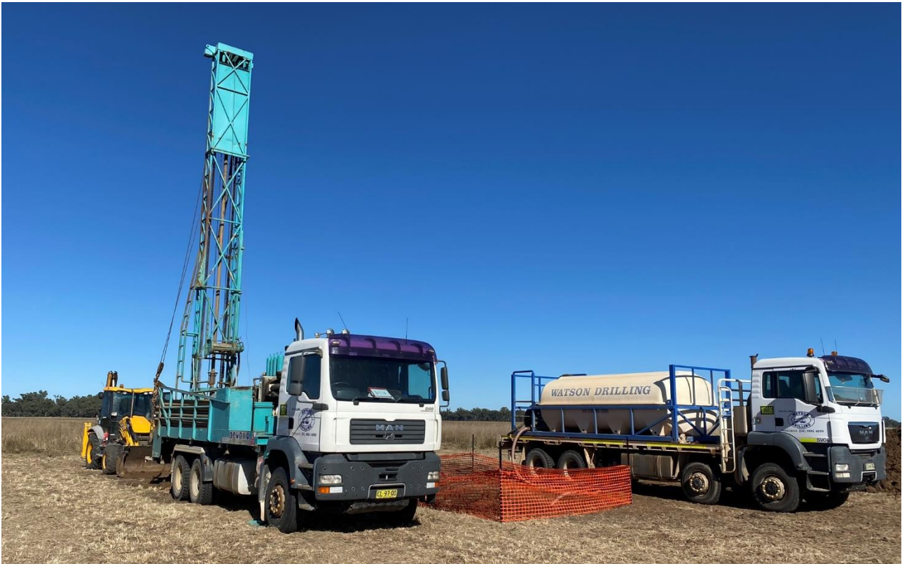
Installation of water bores underway at the Sunrise Project borefield
