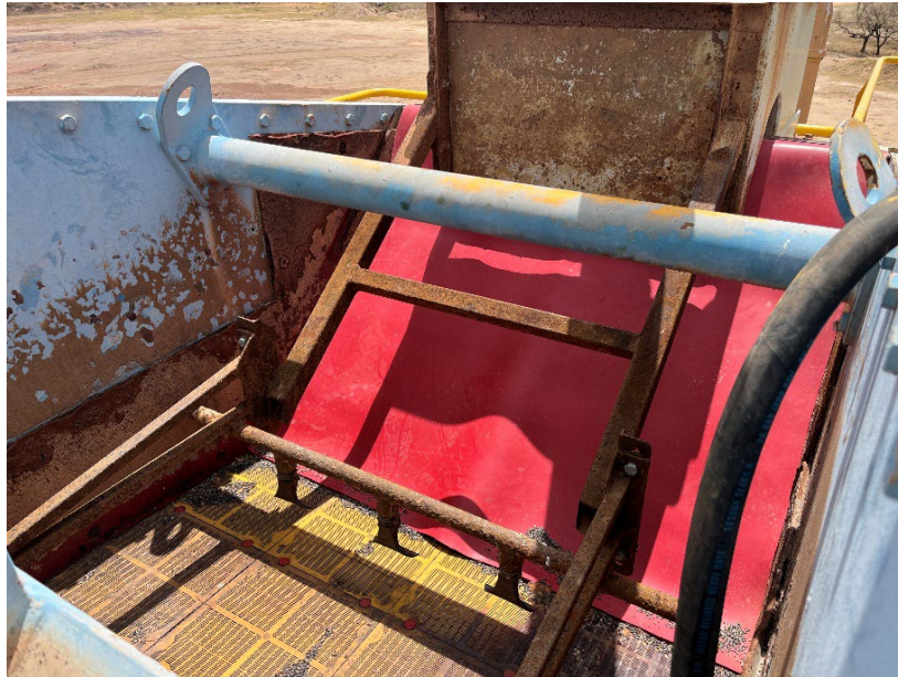
Figure 4: New Linatex installed on the Trash screen on top of Tank 1
