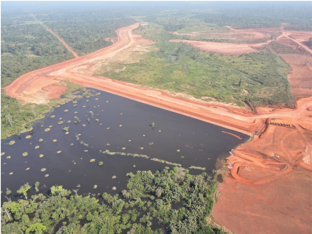
Figure 9: Water storage dam and diversion channel
