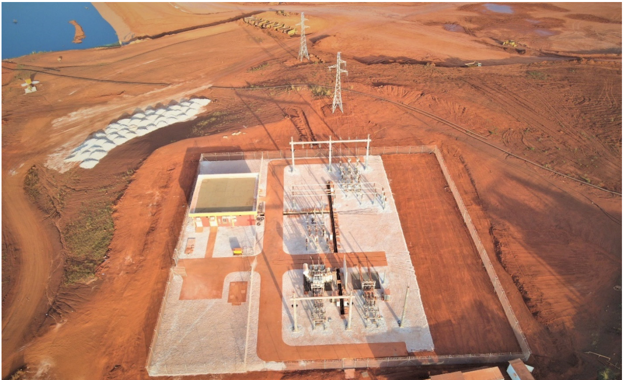
Figure 10: Abujar 90kV substation
