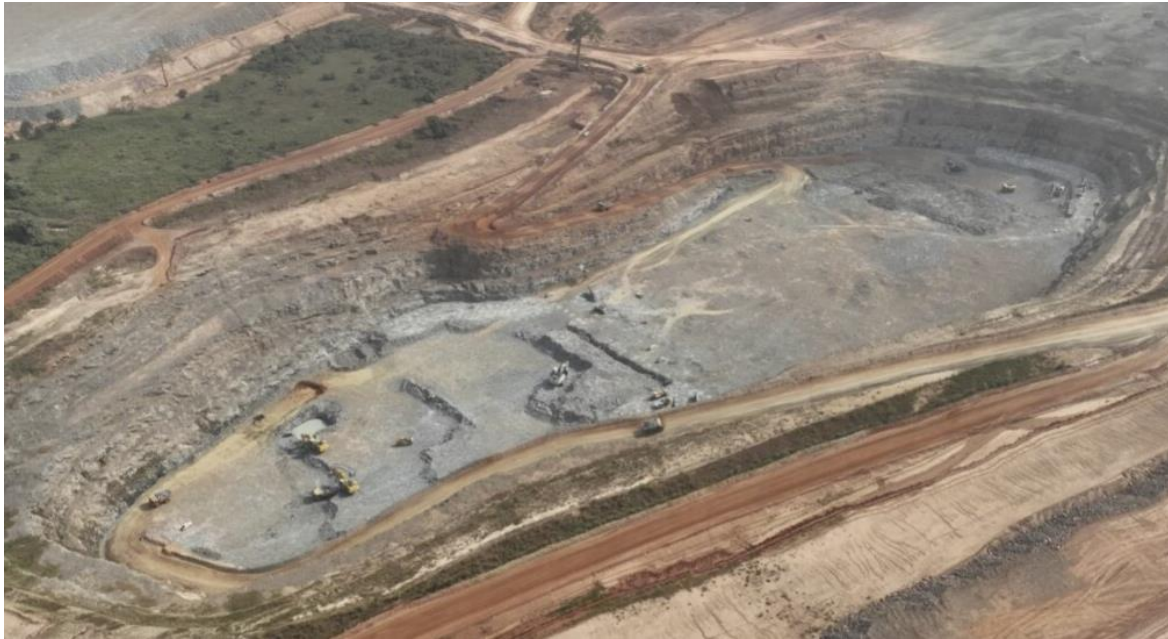
Figure 2: AG Main Pit Development at Abujar Gold Mine
