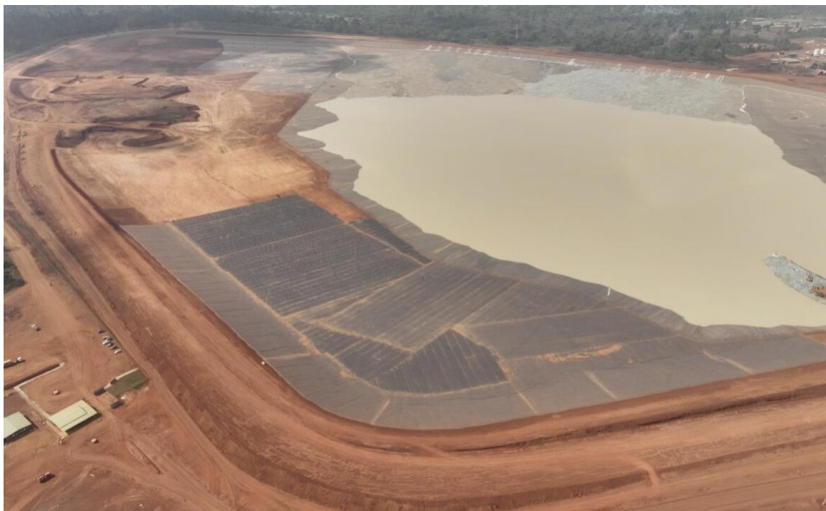
Figure 1: Tailings Dam expansion works at Abujar Gold Mine
