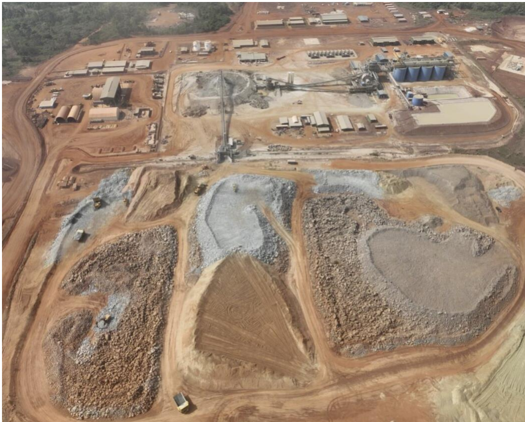
Figure 3: Process plant and ROM Pad at Abujar Gold Mine
