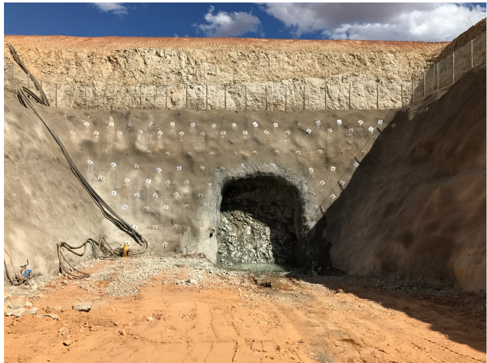
Figure 1: Construction of the new Monty decline.
