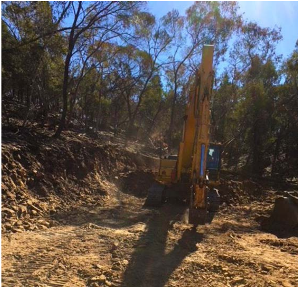
Figure 2: Drill site preparation – Blind Calf Prospect, Lachlan Cu-Au Project
