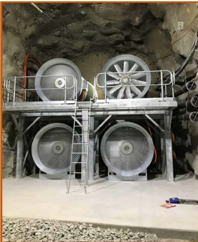
Figure 1: Monty primary ventilation fan installation
