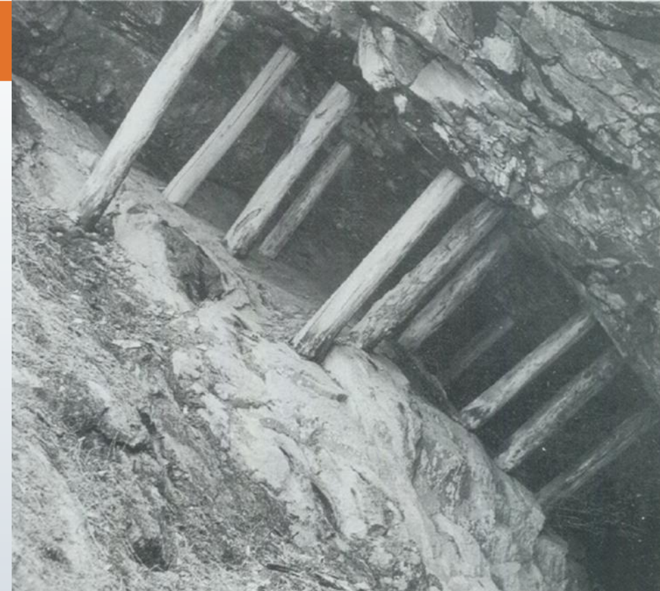
Historically mined mineralised shear zone at Storgruvan
