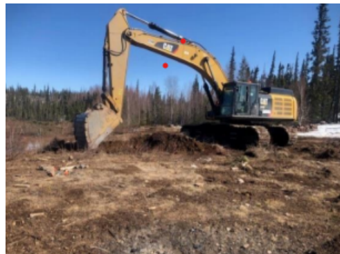
Figures 1 and 2 - Excavating the ore sorter location; Loading cobble to bring to ore sorter pad
