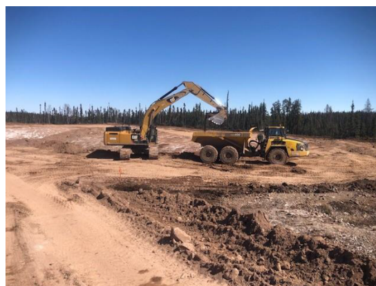
Figure 8 – Loading overburden
