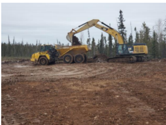
Figure 7 - Loading till from north-east side of North T pit
