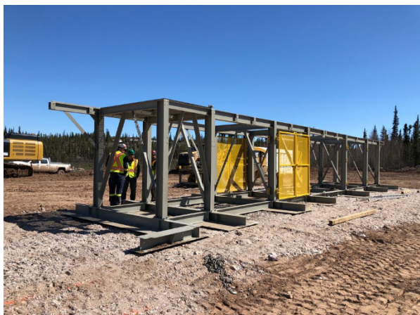
Figure 5 and 6 – Ore sorter frame located in position and ore sorter awaiting placement
