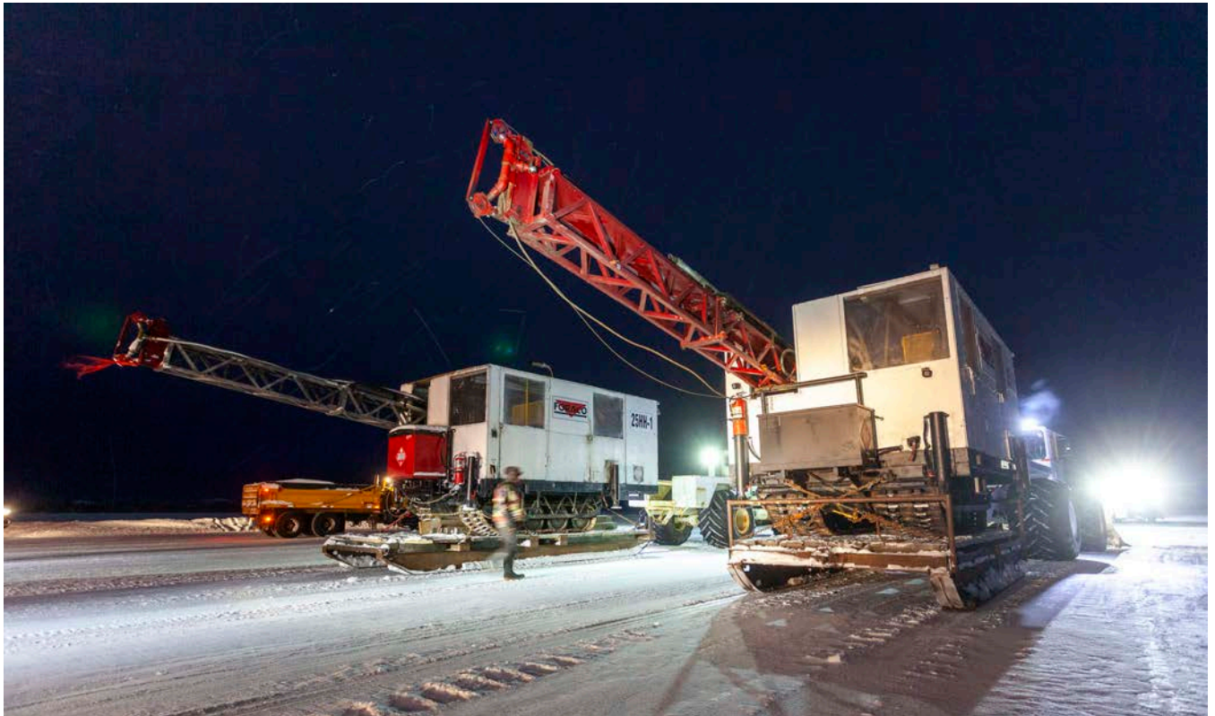
Figure 1: Mobilisation of Drill Rigs (February 2023)
